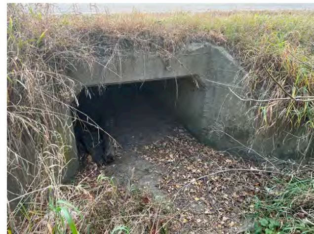
Photo 18: Culvert and Ephemeral stream 1, facing west.
