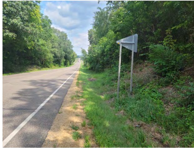
Photo 4: Edge of Roadside Ditch 1, facing south.
