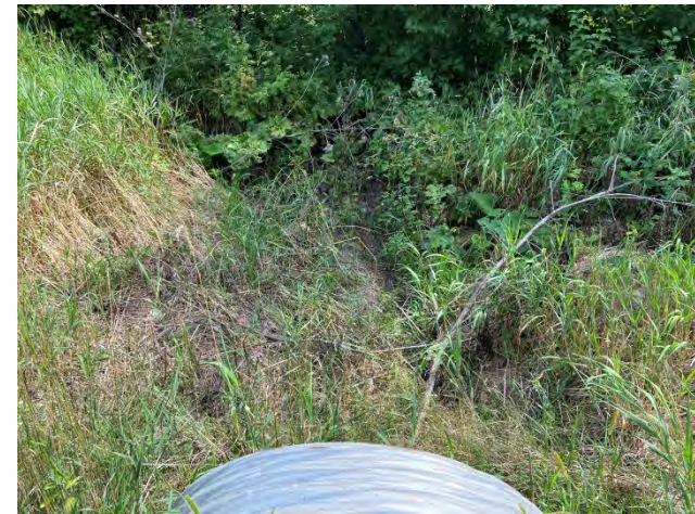
Photo 11: Culvert and Ephemeral Stream 1, facing east.
