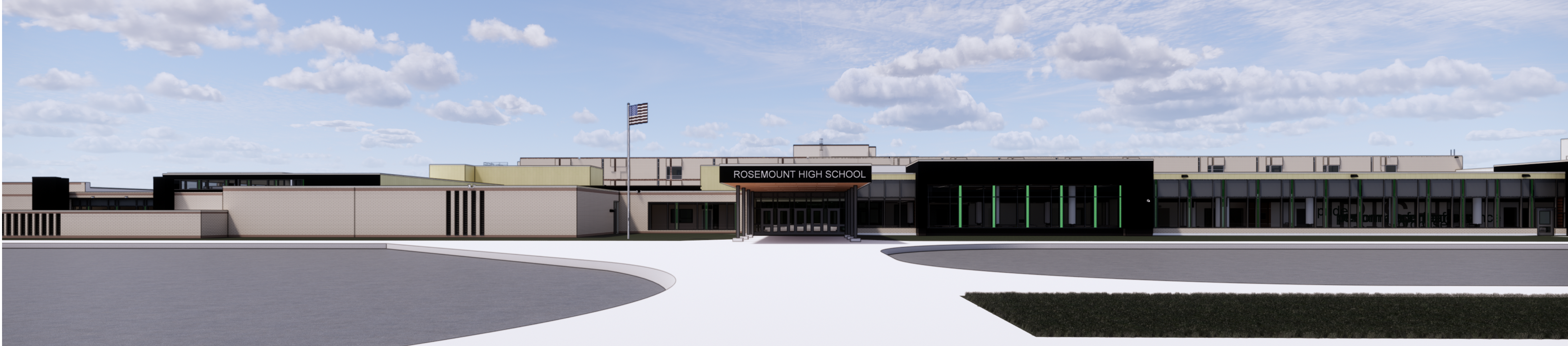
VIEW OF MAIN BUILDING ENTRY
