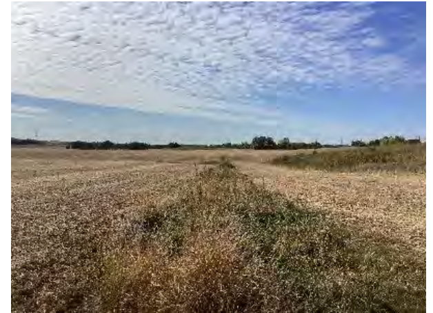
Photo 6: Grass-lined swale, facing west.
